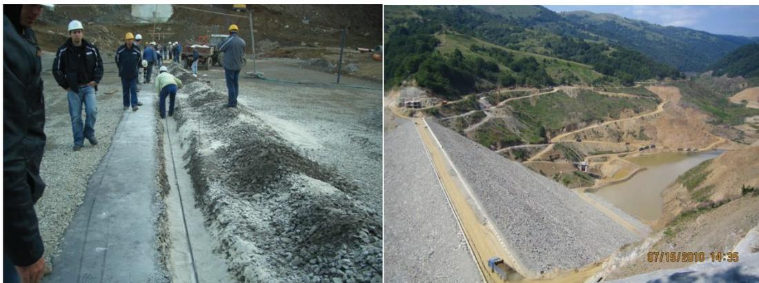
**Figure 8. Knezevo rock fill dam in Macedonia installation of the FO cables (left side)**
