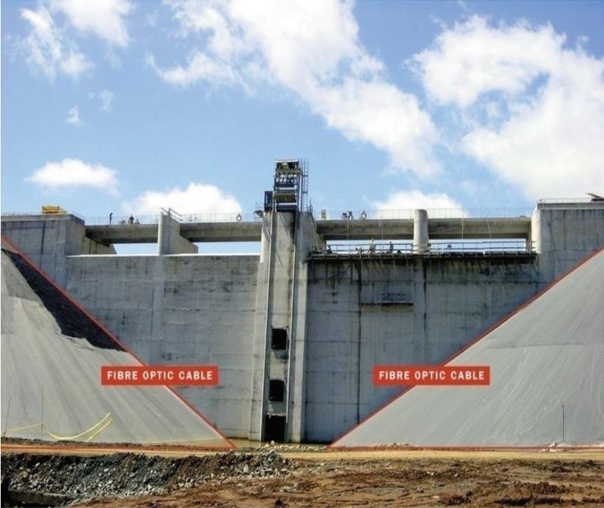
Figure 6. Fibre optic cables installed at the Midlands dam in Mauritius
