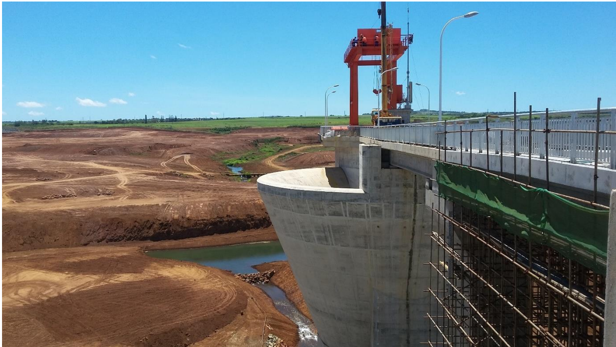
Construction of the Bagatelle Dam
