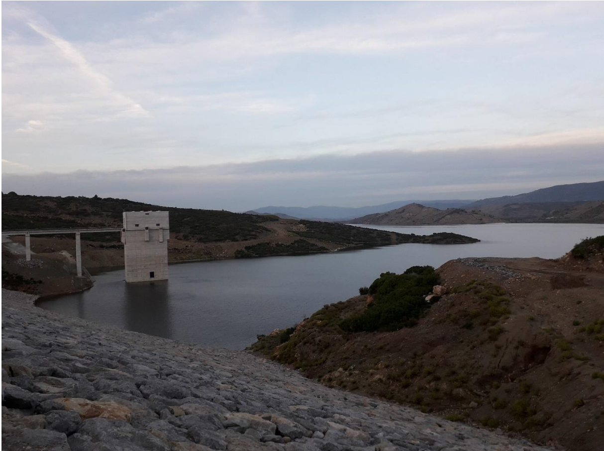
Dar Khrofa Dam, Morocco
