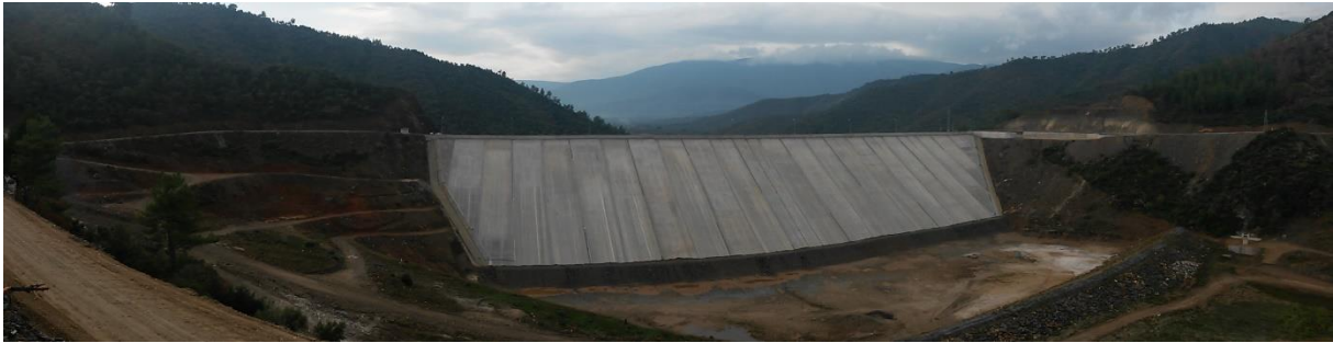
Upstream concrete face sealing of Derince Dam
