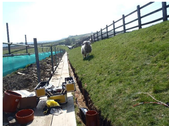
Installation of the fibre optic cable at the Digley Reservoir Embankment
