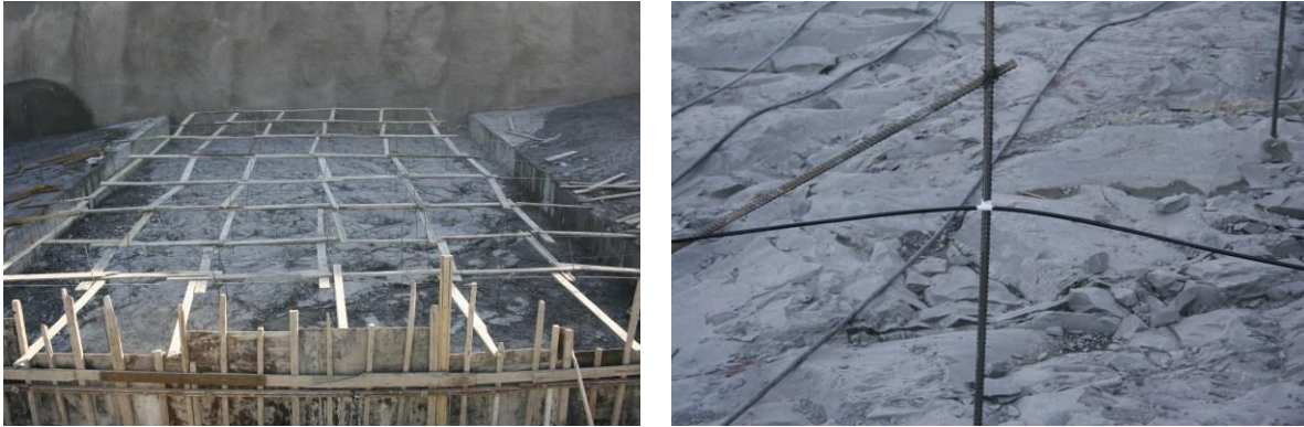
Fixing the fibre optic cable to auxiliary constructions
