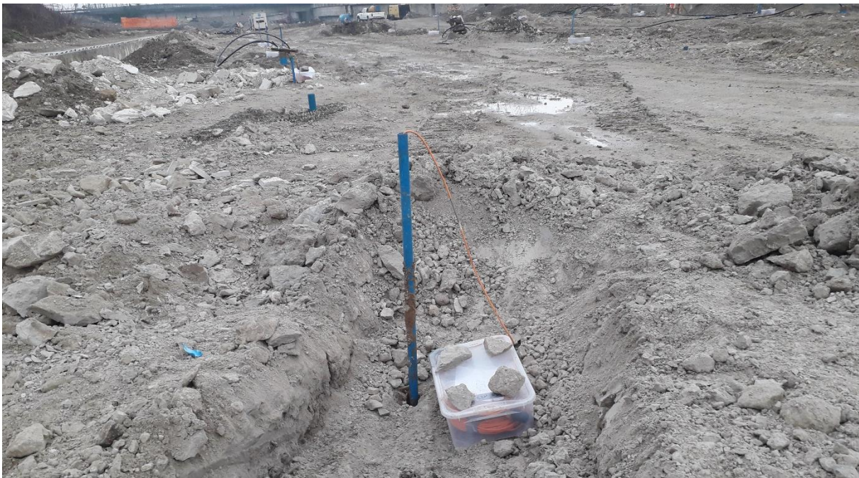
Temperature sounding with data logger
