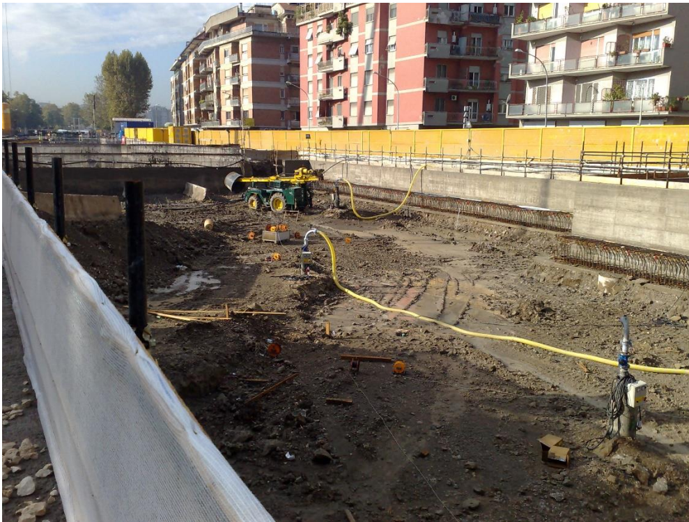
Construction site Conca d'Oro Metro B1 in Rome, Italy
