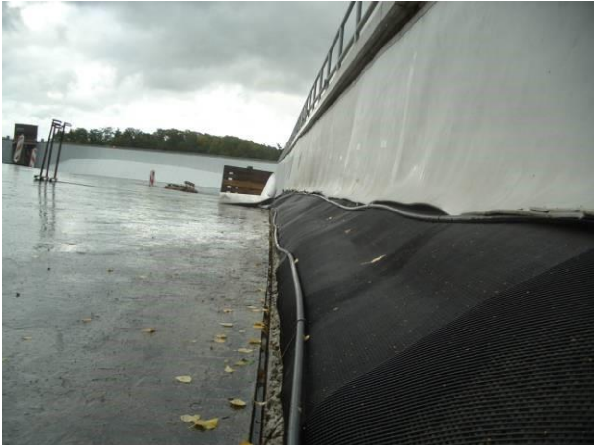
Installation of the fibre optic cable along the geomembrane
