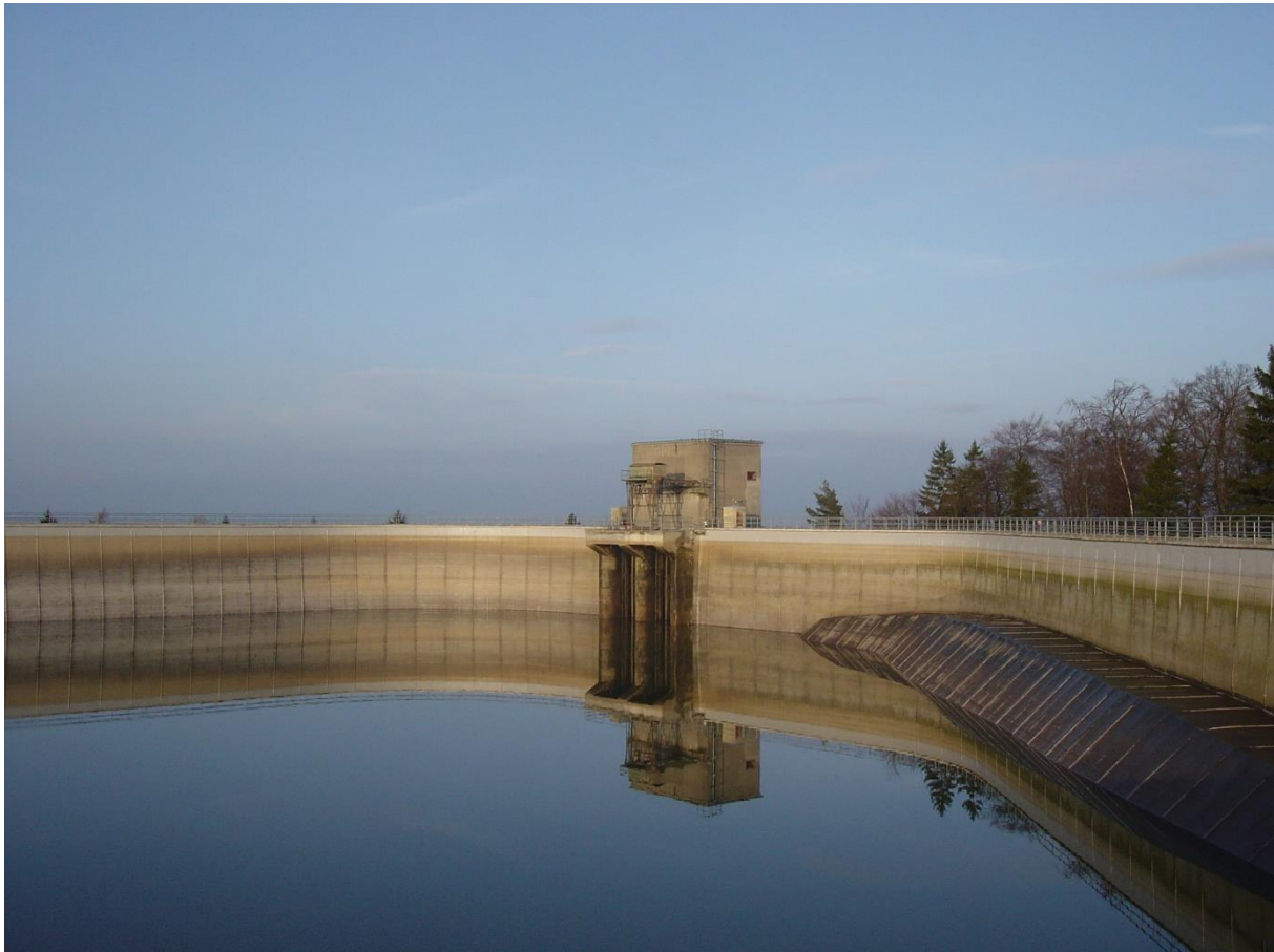
Pumped storage power plant Waldeck I, Germany
