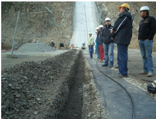
Cable installation
