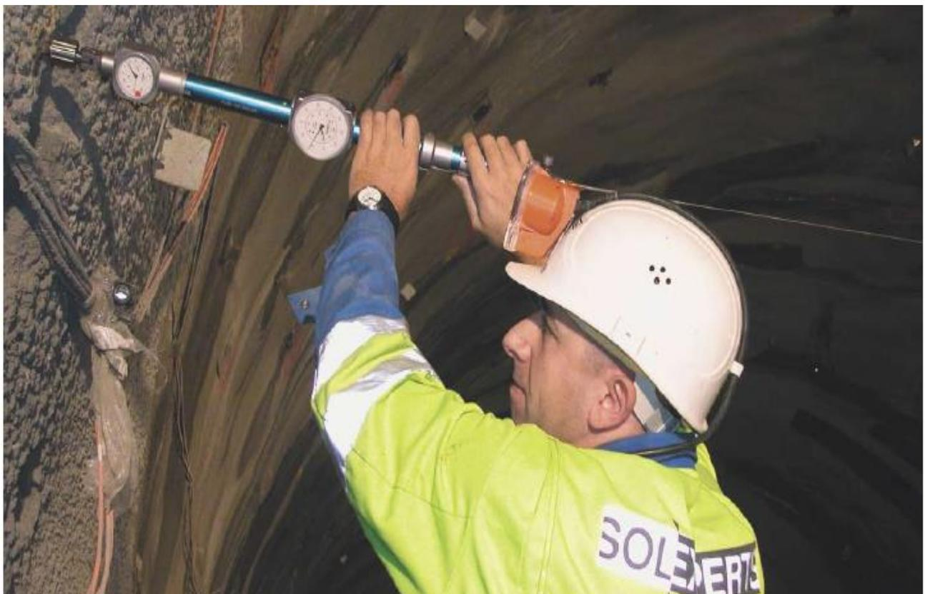
*Figure 2.26 shows the installation of distometer in tunnel.*
