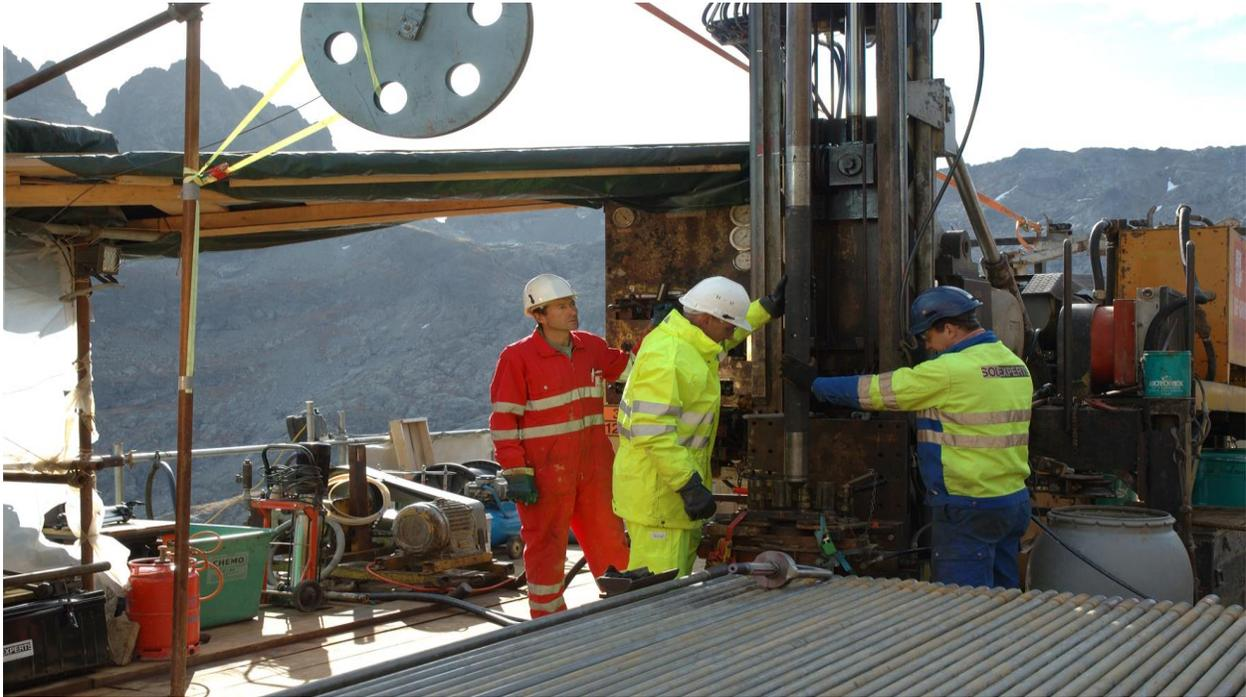
***Figure 2.35 Installation of the dilatometer probe in exploratory borehole for Emosson pumped storage hydropower plant (Switzerland) Dilatometer probe, Sedimentation tube and Installation rods.***
