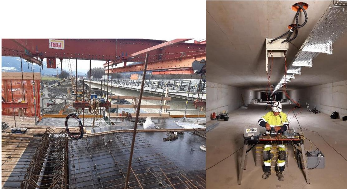
Figure 6: Installation of the fiber optic cables in the structure (left) and splicing of the cables (right)
