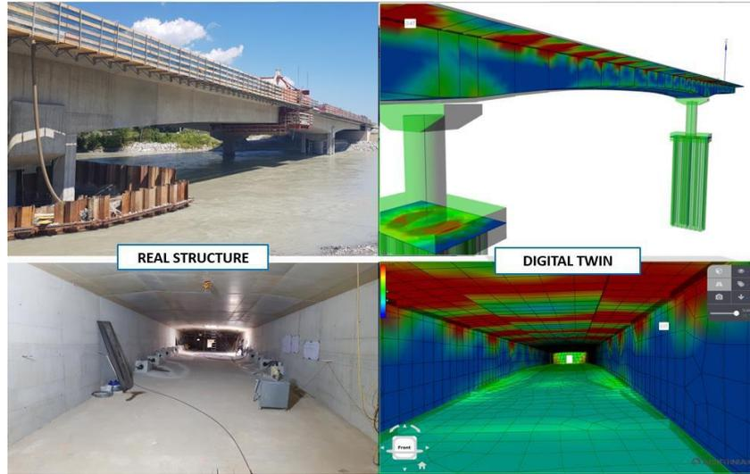
**Figure 1:** Comparison of real structure and digital twin of a highway prestressed concrete bridge.
