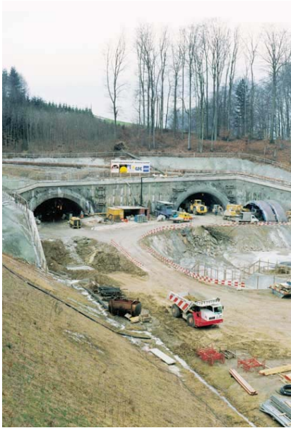
Figure 2.1. Aeschertunnel North Entry
