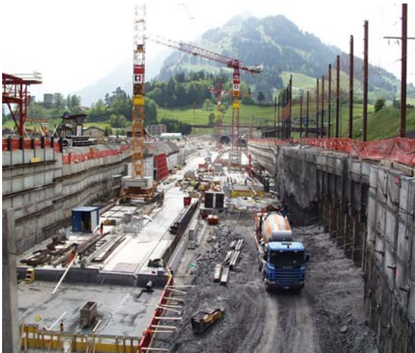
Figure 3.1 Overview of the construction site
