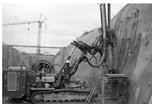
Figure 9. Installation of the micropiles
