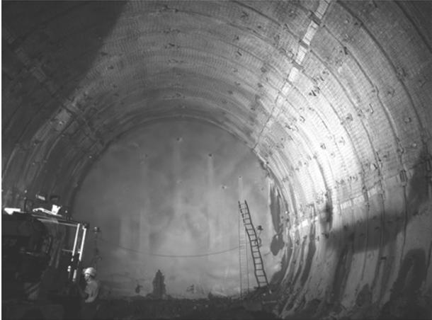
Figure 5: Deformable lining with HDC elements in Lötschberg base tunnel
