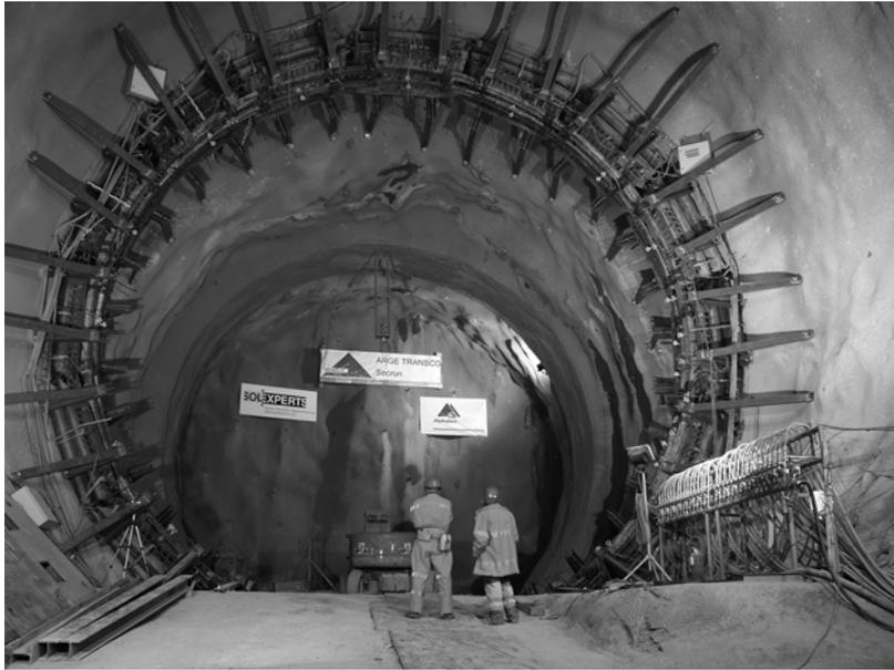
Figure 2: 1:1 In-situ Test of steel arches, Sedrun, Switzerland
