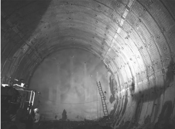
Figure 5: Deformable lining with HDC elements in Löttschberg base tunnel
