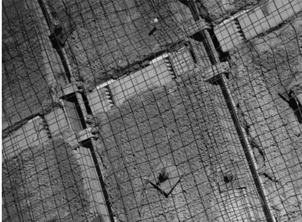
Figure 6: Detail of an installed HDC elements
