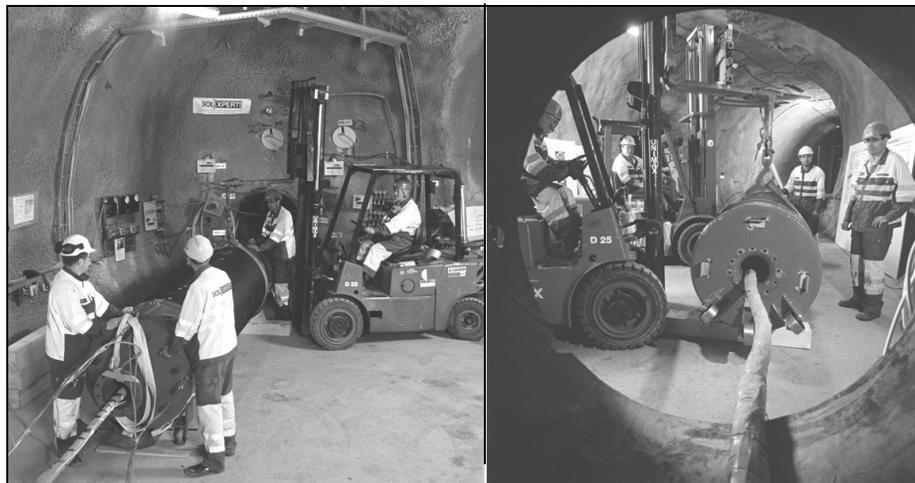
Figure 12: Megapacker before the emplacement into the microtunnel. Cables and lines pass through the megapacker centre pipe; source: COMET Photoshopping GmbH.
