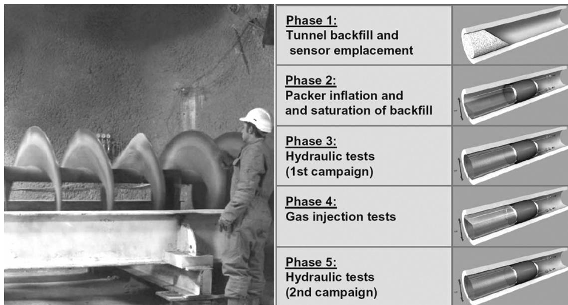
Figure 3: Excavation of the microtunnel with an auger rig (Phase 0) and general test plan of the HG-A experiment; source: Mont Terri Consortium.
