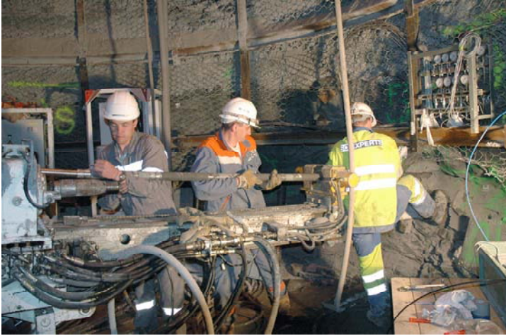
Photo 1: MMPS Installation in a borehole
