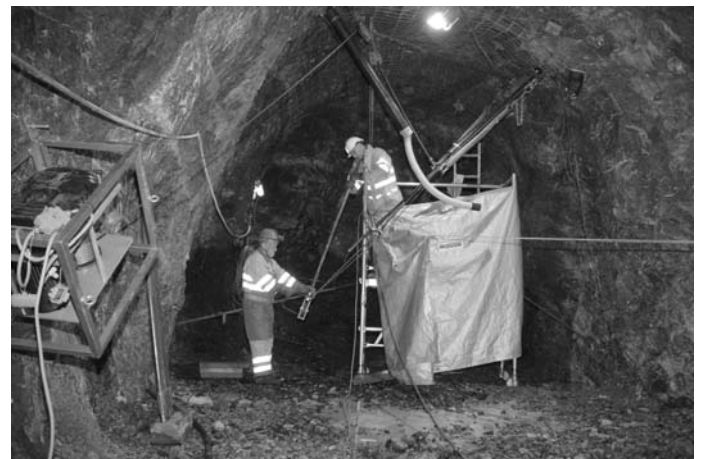
Figure 4. Installation of the dilatometer probe.
