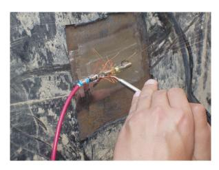
Fig. 15 Installation of vibrating wire gauges on a high-pressure gas pipeline in a landslide area
