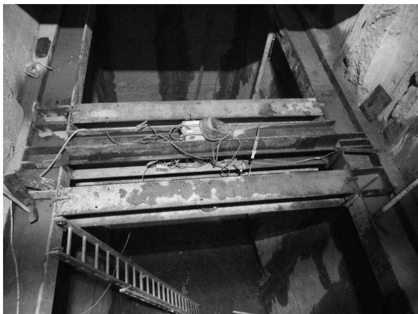
**Figure 10** Additional struts on the left and the right side of the originally planned single strut, the new struts were also instrumented with strain gages
