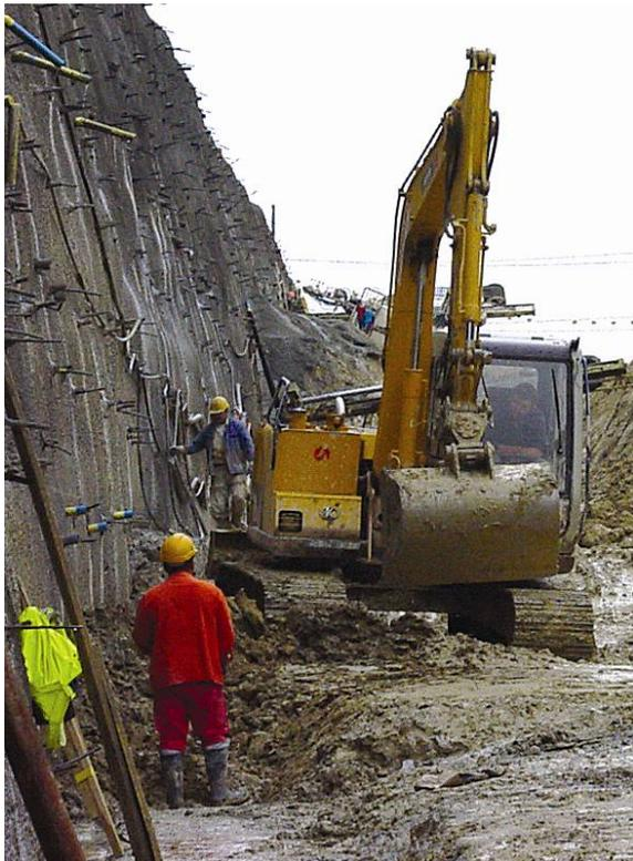
**Abb. 7.9:** Messanker Önzbergtunnel
