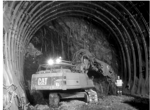
Figure 3. Appearance of the Carboniferous rock mass during excavation. Chainage 1350 m.
