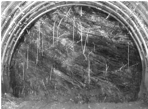
Figure 2. Appearance of the Carboniferous rock mass at the face. Chainage 1414 m.
