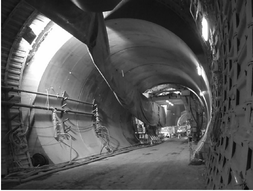
Figure 10. Concrete lining installation.
