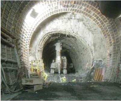
Above: View in the background of the support system initially adopted which underwent convergences up to 2m and later needed to be re-profiled
