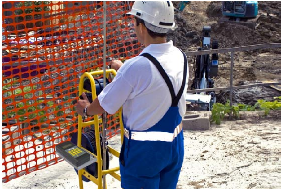
Sliding Deformer and Sliding Micrometer measurement with the MRD
