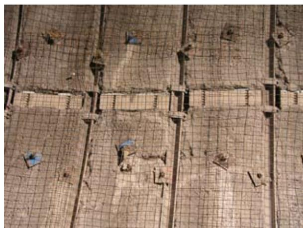
Fig. 10: Highly compressible concrete elements inserted in the shotcrete lining
