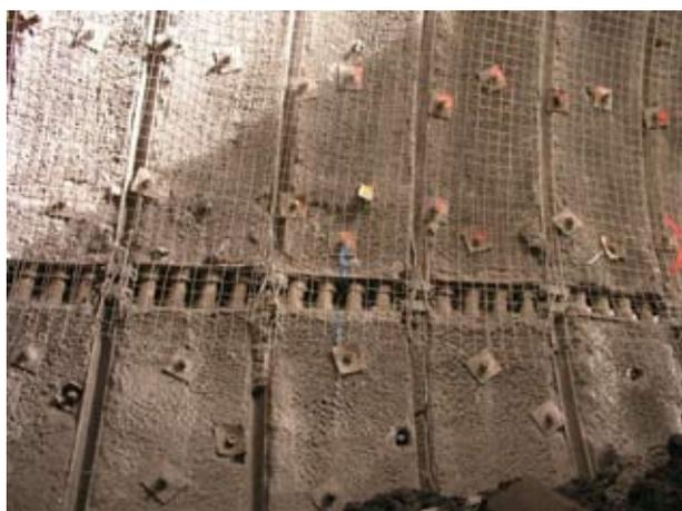
Fig. 9: Steel cylinders inserted into slots of the shotcrete lining
