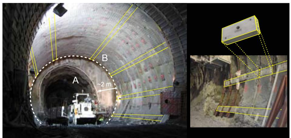
Fig. 15: Lyon-Turin high speed rail link, access adit: convergence up to 2 m (Profile A), Re-profiling and application of yielding concrete elements (Profile B)
